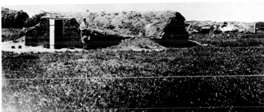
Figure 15: Roof thatched with straw dipped in clay mix. A dug-out type of home in early 1900's.
